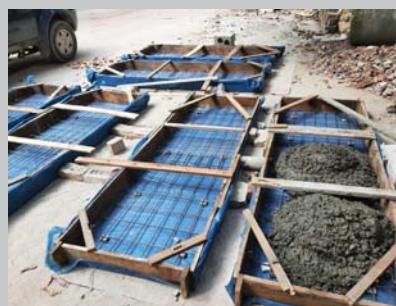
Figure- Casting of One Way Slab with WWR
