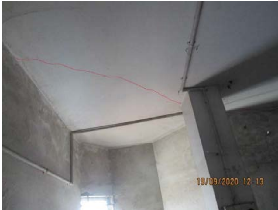
Figure 1(a): Flat plate system structure and diagonal cracks on the ceiling in the cantilever portion
