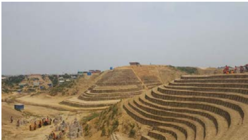
Figure 1.3: Slope protection measure in the locations of Ukhiya (a)close-up view (b)full view
